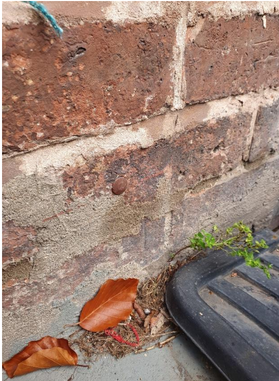
Evidence of historic DPC
